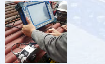
Corrosion Inspection of Boiler Water Wall
